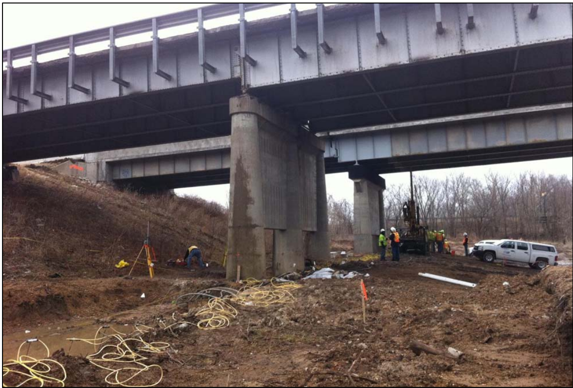
Figure 6.7. Photograph of the study site (looking southeast). ERT data are being acquired on Traverse 3.
